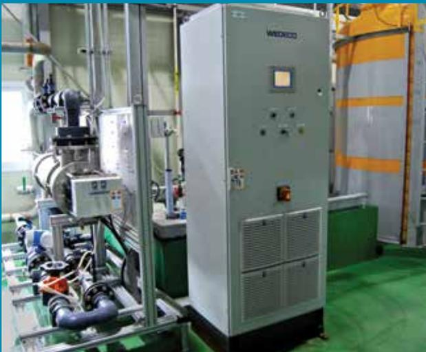
Wedeco MiPro™ photo is delivered skid mounted including all controls and analytical devices like UVT monitor and H<sub>2</sub>O<sub>2</sub> measurement.
