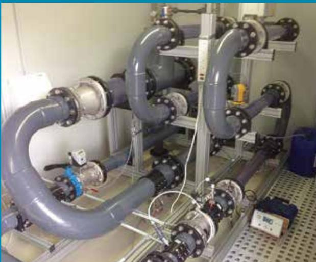
Pro<sub>3</sub> mix utilizes ozone and peroxide to break down pesticides while limiting bromate production.
