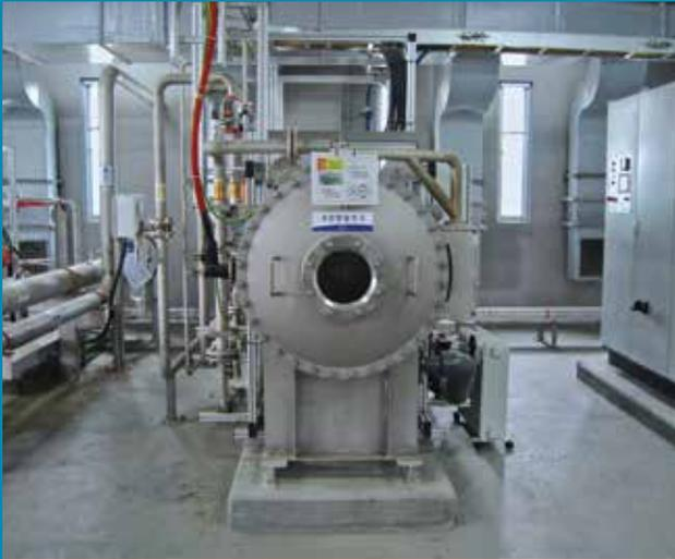
Three Wedeco PDO 1000 ozone generators are producing up to 51 kg of ozone per hour from liquid oxygen.
