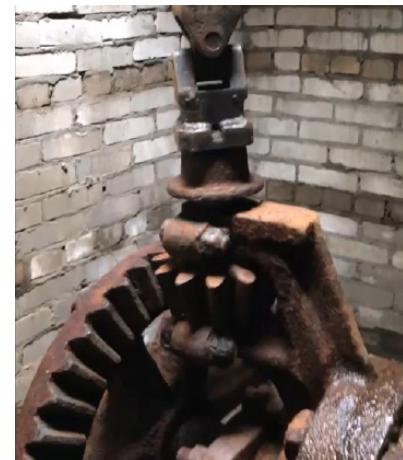
Xylem was successful in quickly rehabilitating this inoperable 87-year old Clow Gate valve.
