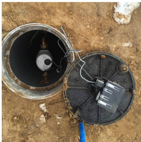
A Sensus iPERL meter connects to a SmartPoint to gather data for the utility.
