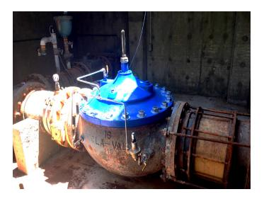
The Water Authority has hundreds of pressurereducing valve sites across the service area that can now be monitored with the batterypowered Smart Gateway Sensor Interface for timely remote management. Issues can be resolved within hours rather than weeks.
