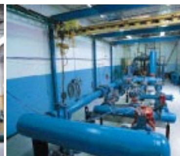
High Pressure Flow Loop; up to 62 bar (900 psi)
